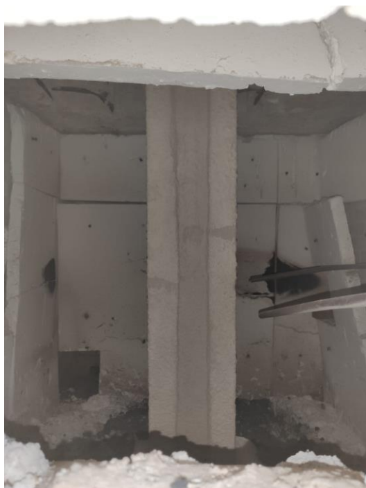
Photo №1. Girder before testing
